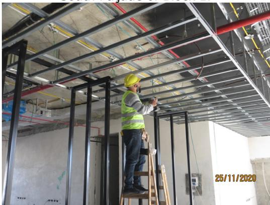
False ceiling works ongoing on the ground floor of Block 1 during November 2020.
