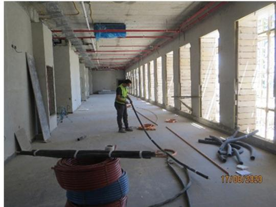
Celling Mechanical and Electrical first fix ongoing in Block 1 August 2020.
