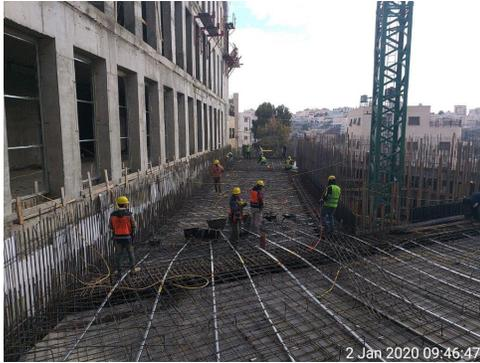
Roof slab reinforcement and shuttering works in Block 4.
